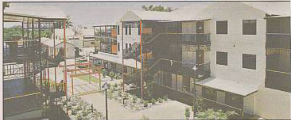
Shiba Lane uses Lysaght Custom Orb profile cladding in a heritage setting. storey building there were no suitable cranes available.
